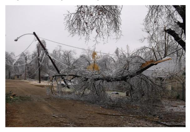
Figure 2-58: Downed power line during the 2013 ice storm in Paris, Texas.<sup>330</sup>
