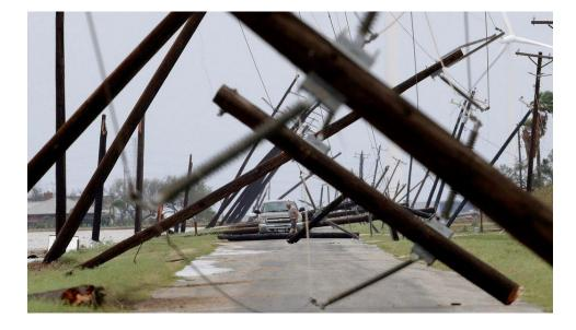
Figure 2-30: Downed utility lines near Taft, Texas, during Hurricane Harvey.<sup>121</sup>
