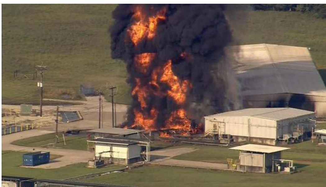
Figure 3-67: Arkema chemical plant explosion in Crosby in 2017. 404
