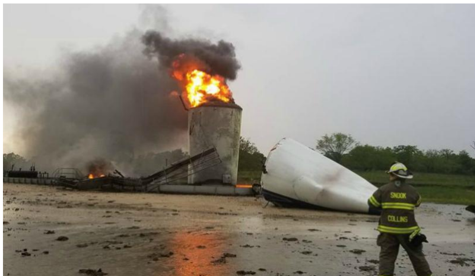
Figure 3-63: Lightning ignited oil tanks in Burleson County in 2018. 353
