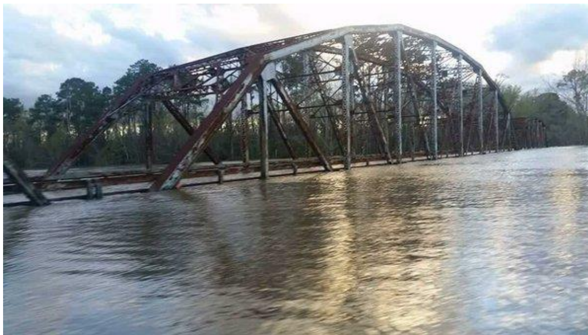
Figure 3-4: Burr’s Ferry Bridge SH 63 over the Sabine River 11
