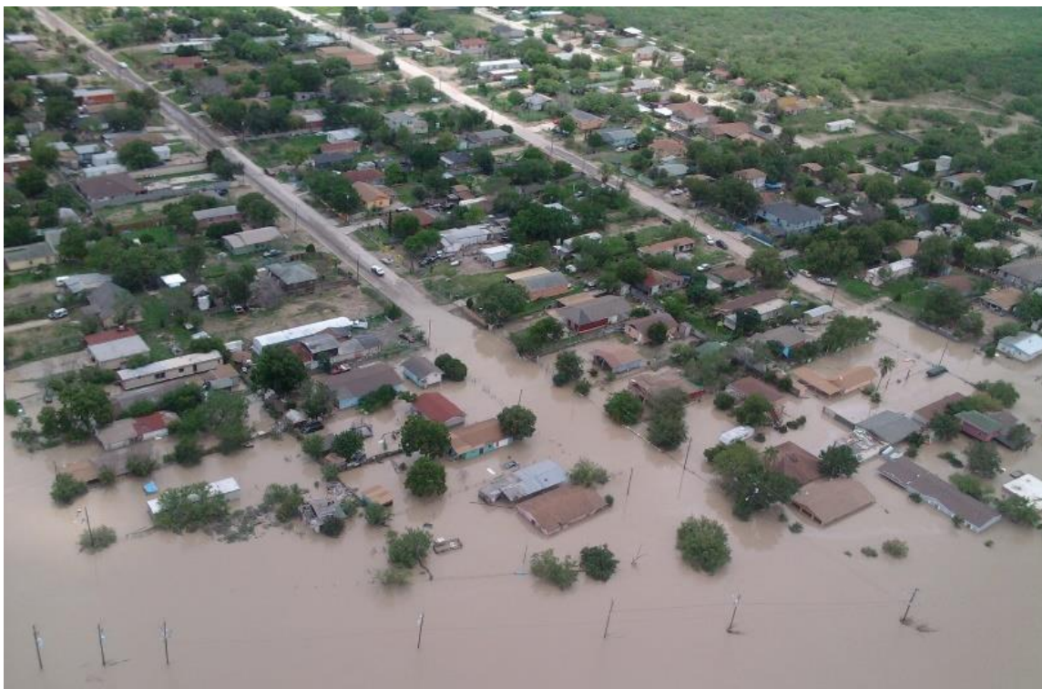
Figure 3-36: Laredo, Texas, during 2010 Flooding. 144
