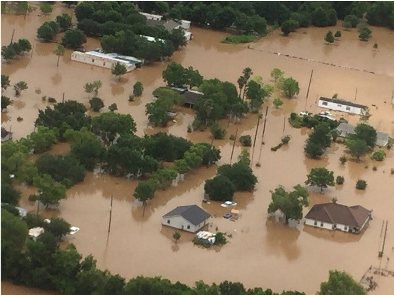
Flood Damage in the Houston Region on June 3, 2016 – Photo Courtesy of Twitter.com/GregAbbott_TX
